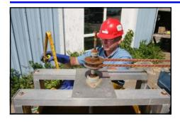
Record level in mix tank and subtract amount from previous volume to attain gallons of slurry processed in first phase fill.
