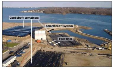
About 26,000 cubic yards of sediment were hydraulically dredged from the bottom of the harbor. Approximately 2,000 linear feet of pipeline conveyed
