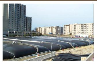
Impacted sediments from the Geotube® containers were blended with on-site soils and imported fill. More than 100,000 cubic yards of soils and sediments were mixed on-site and spread as backfill to achieve preconstruction grade.
